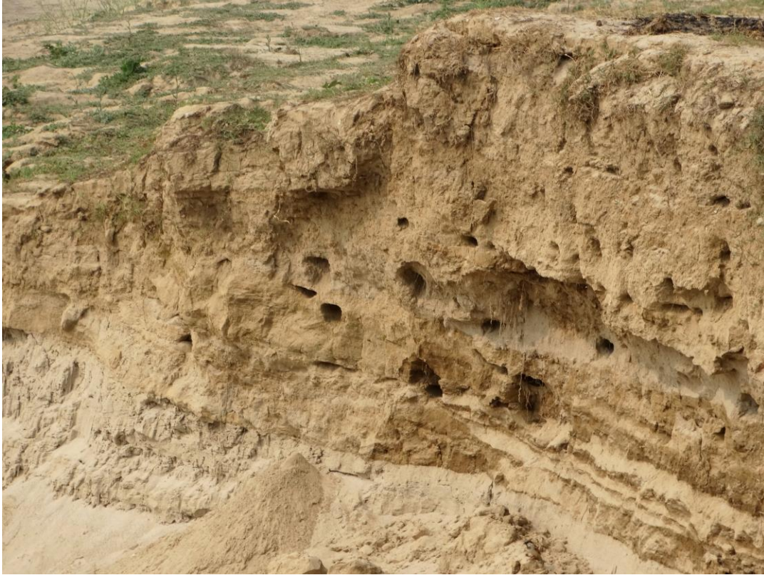
Image 58 : Lateral Bank Erosion As Observed Near Maldepur
