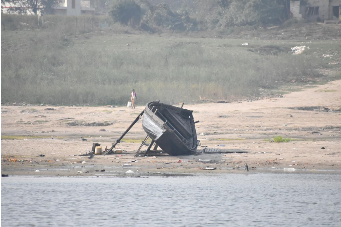
Image 64 : Construction Of A Big-Sized Mechanized Wooden Boat For Transportation Near Ujjiar Ghat In Ballia Distt.
