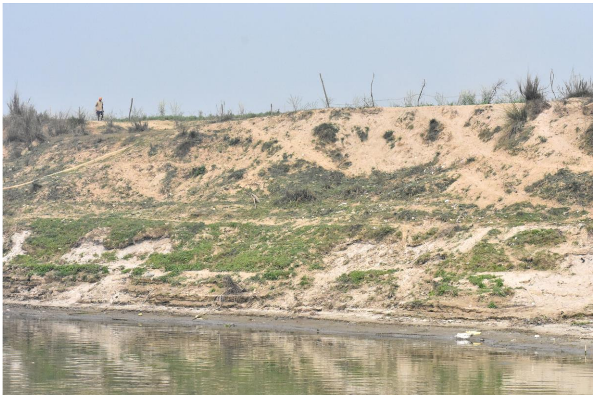
Image 61 : Bank Erosion Prone Site Near Daya Chhapra
