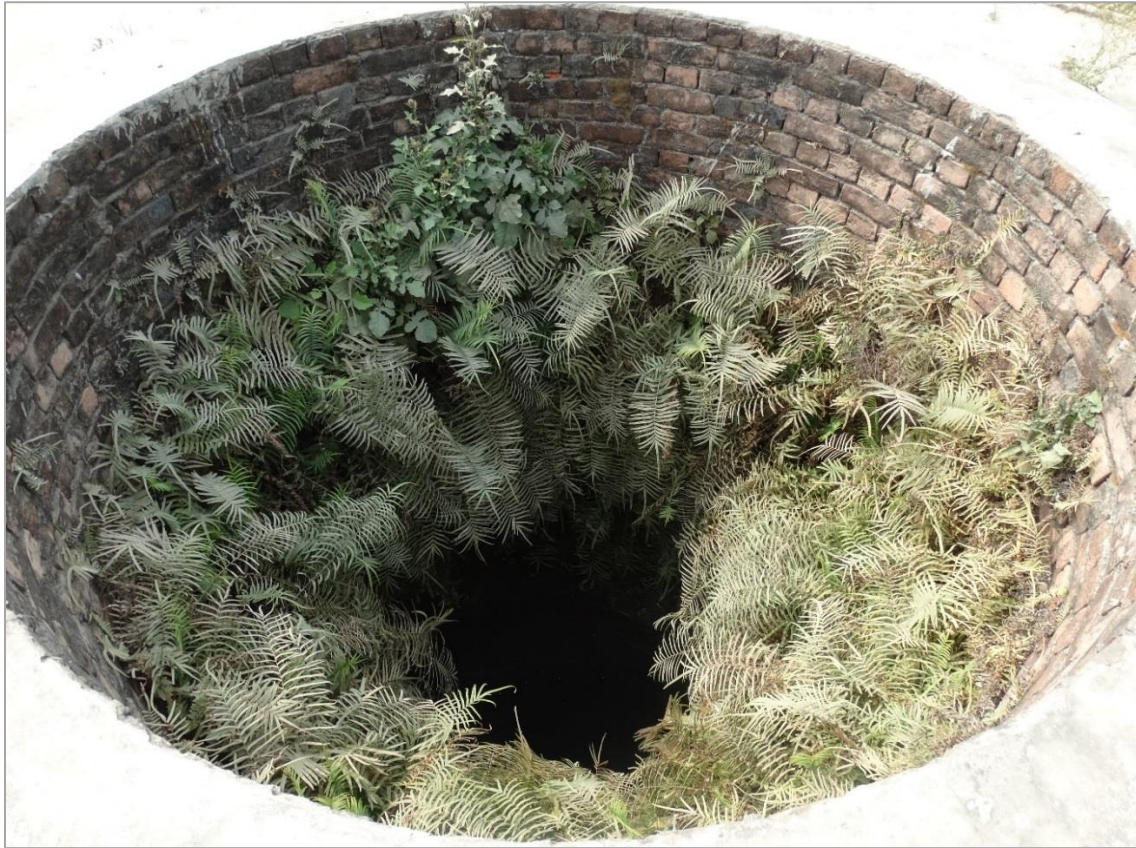
Image 55 : Inside Photo of the Well. Ferns And Other Vegetation Growth Has Taken Over
